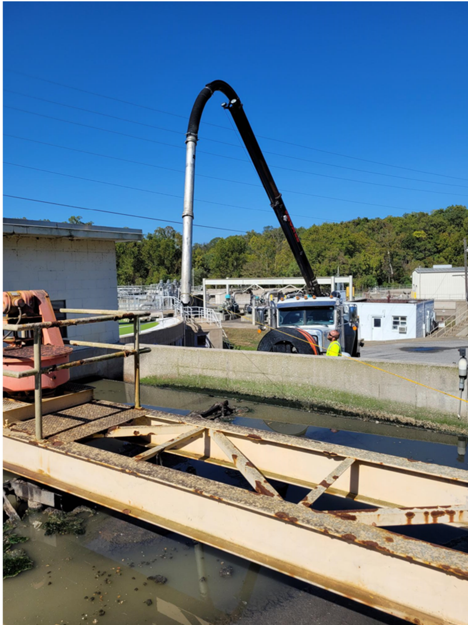
Existing Grit Basin cleaning on October 15, 2025
